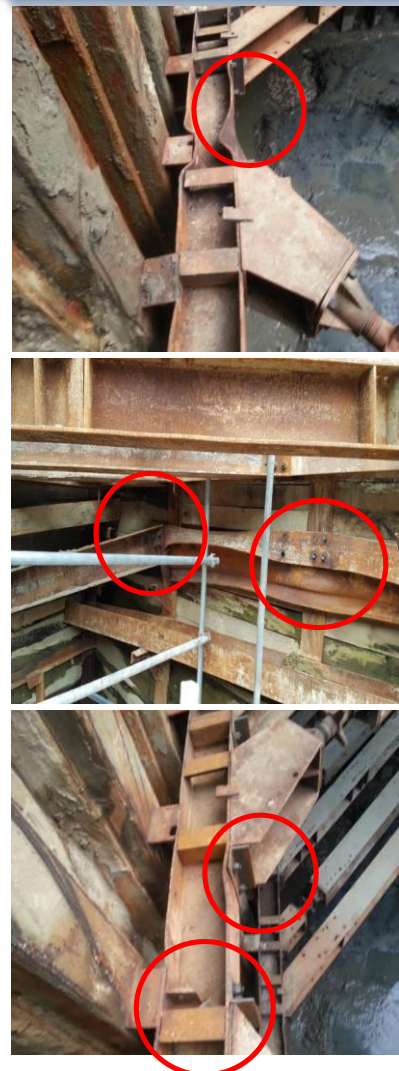
[Photo] Waling Deformation Cases
